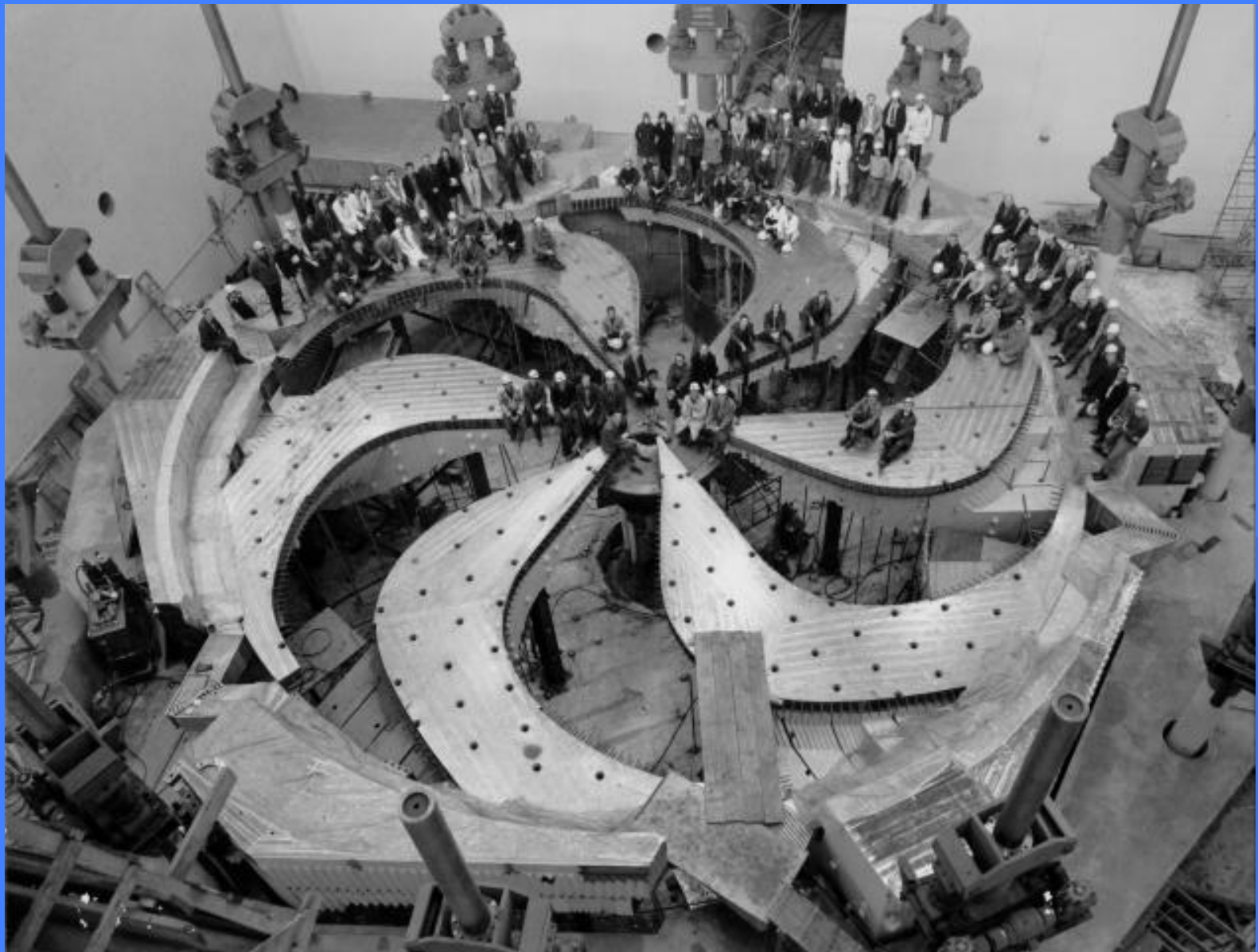
Worlds largest cyclotron - 500MeV protons at up to 200\mu\text{A}
