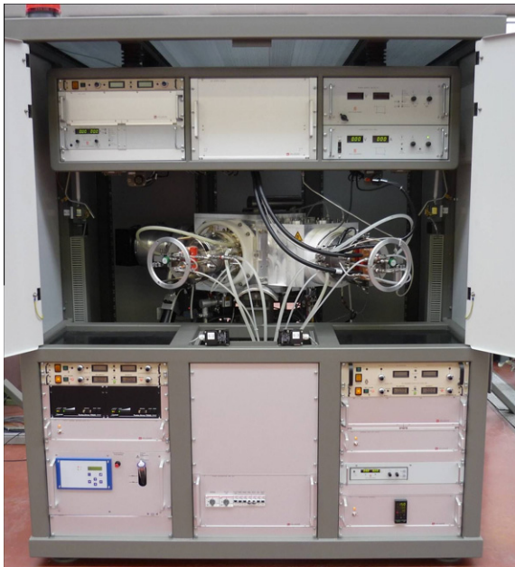
Fig. 1. Front view of the dual-source multicusp injector enclosed in cabinet.
