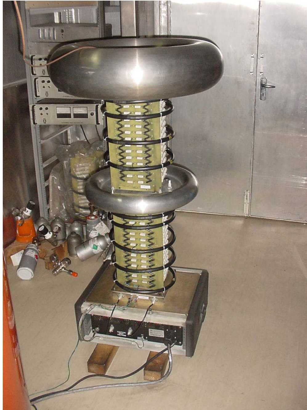
High Voltage Power Supply for biasing the platform
